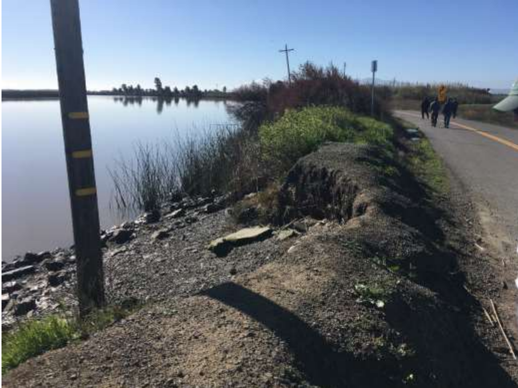
Photo 8 – Levee Adjacent to Island Slough Fishing Pier
