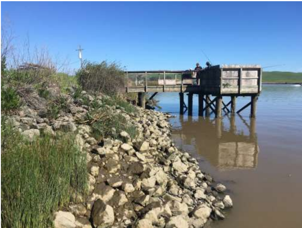
Photo 2 – Island Slough Fishing Pier and Supporting Levee
