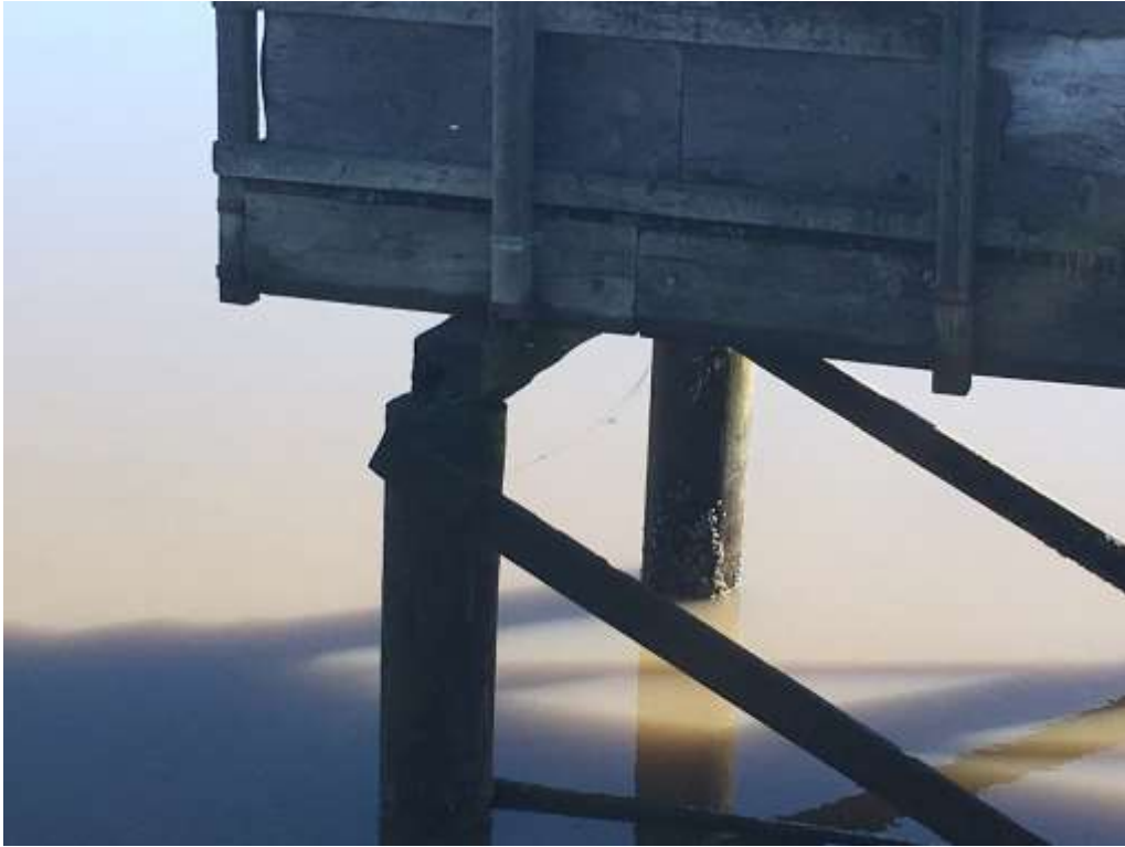
Photo 3 – Island Slough Fishing Pier In-water Support Structure
